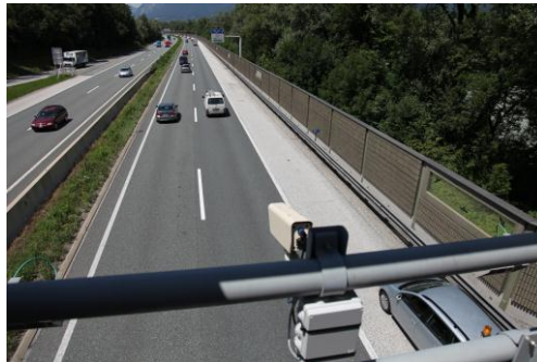
Figure 7: Smart camera mounted on a gantry on Austrian motorway A12
